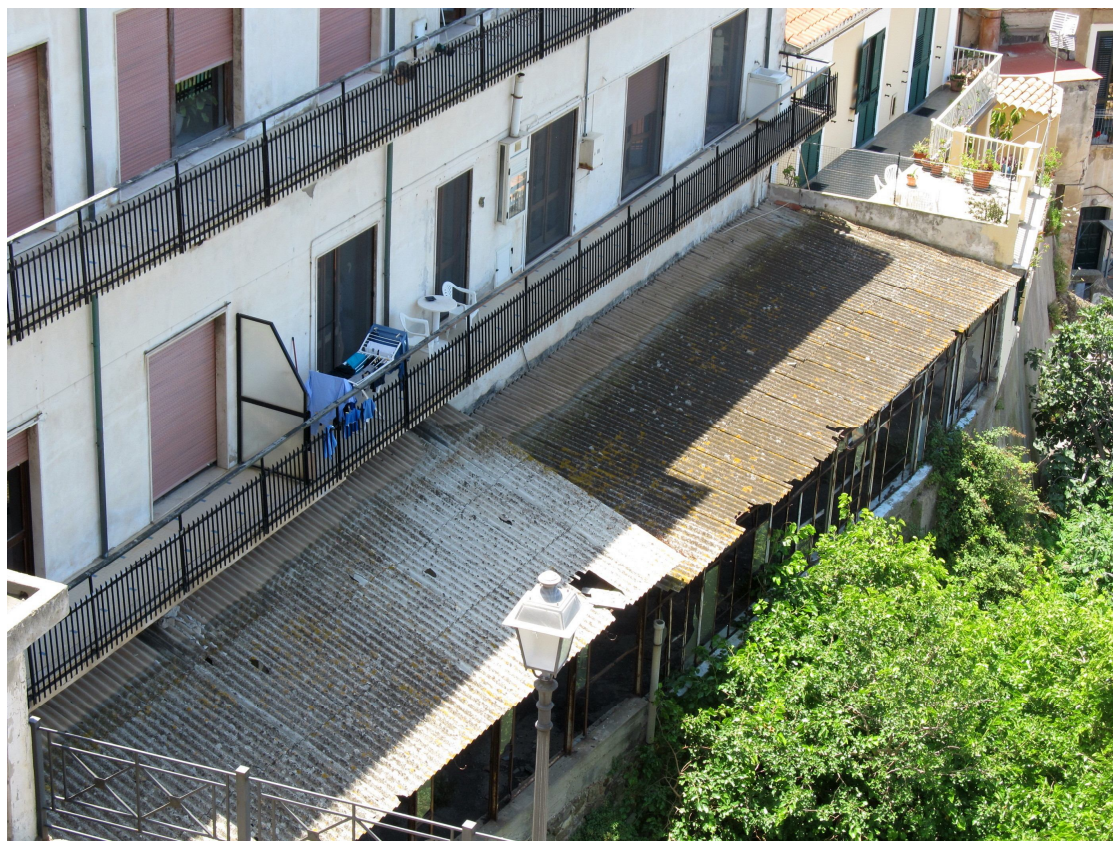
Coperture in eternit
